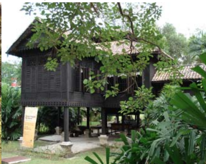
Rumah Penghulu after restoration
