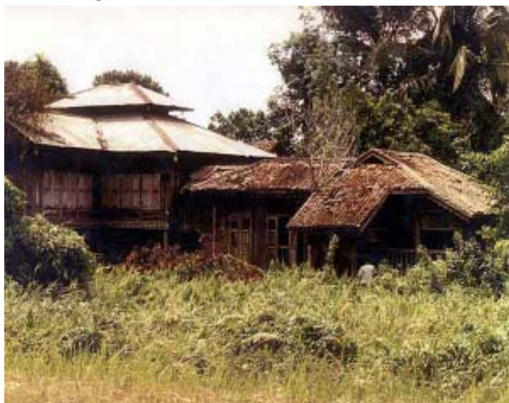
Rumah Penghulu before restoration
